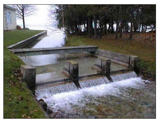
Tressler Dam (North Manistique Lake) at low flow with all boards removed.
