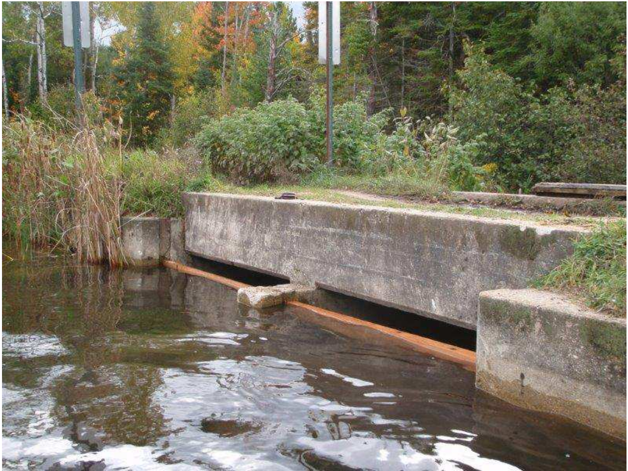
Photo 2. Water Control Structure/spillway 2014 following board maintenance.
