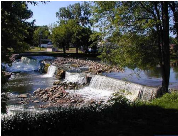
Chesaning Dam breached 2005
