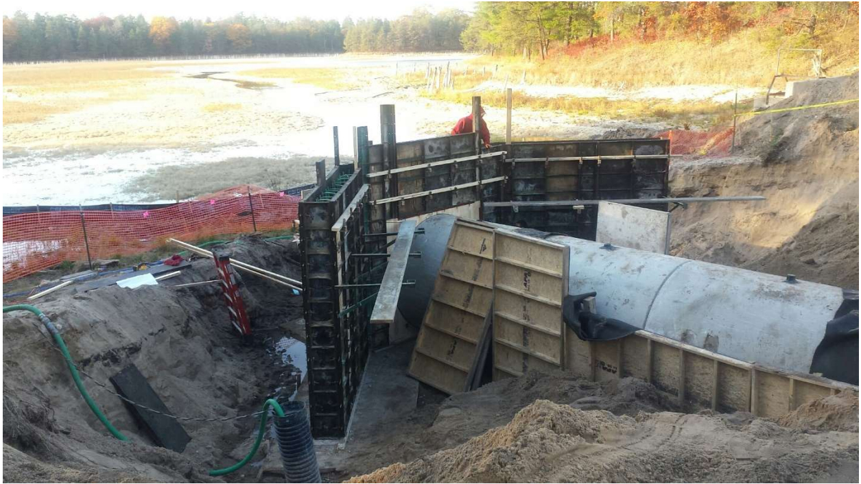
Photo 3. Foch Dam control structure under renovation in 2016.
