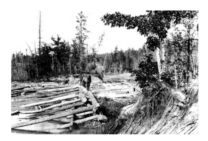
A "cut-off", areas where the river made a large U-shaped bend. The loggers, who systematically removed all the woody debris from the stream channel to facilitate floating logs to market, cut through these bends. This straightened the river and eliminated bends where log jams typically occurred. This photograph is thought to be at the present day site of the US Forest Service Peterson Bridge (M-37) campground on the Pine River, formerly the South Branch of the Manistee River.
