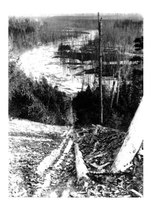
A log sluice located at Udell Hills Rollway in Manistee County, T22N, R15W, Section 36, that is at the mouth of Pine Creek. This method of delivering the logs to the river was more commonly used on the west coast. White rollways, as depicted on the cover photograph, were typical of Michigan's loggers.
